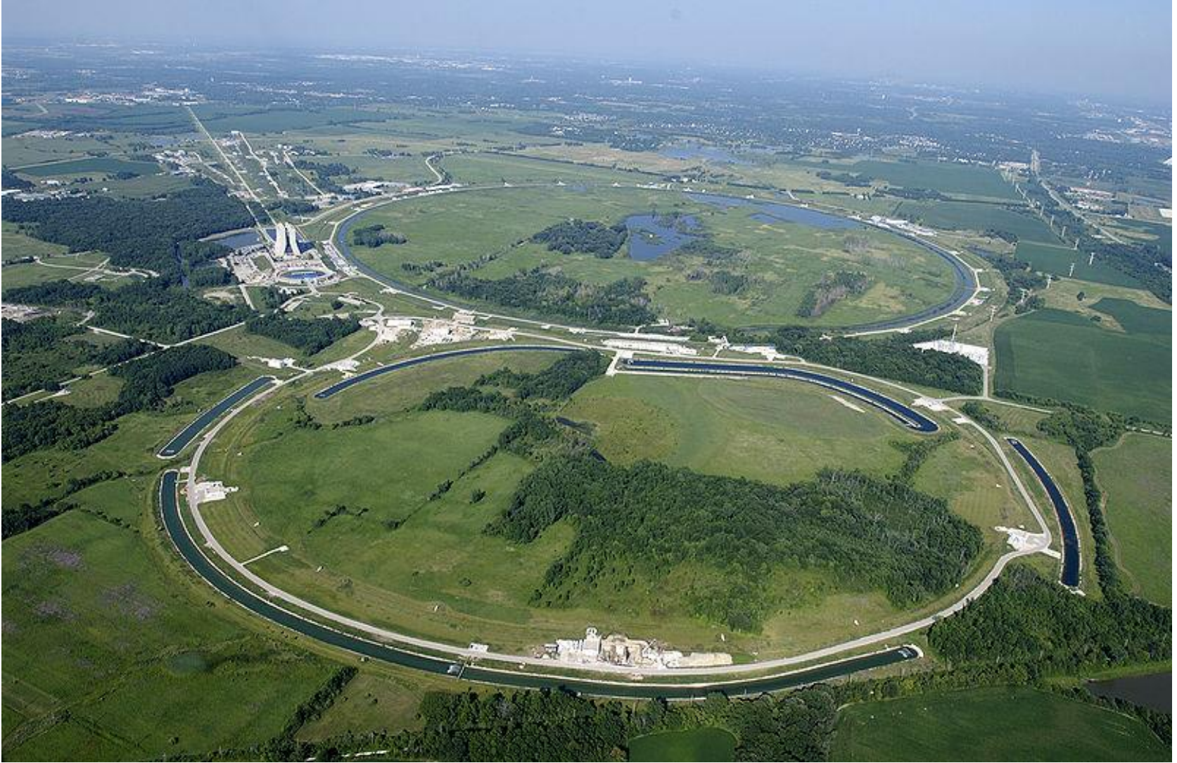
Tevatronul Fermilab (Fermi National Accelerator Laboratory)-SUA-Chicago
